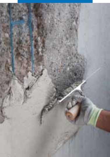
Application of Planitop Smooth & Repair with a spatula
