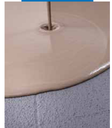
Application of self-levelling smoothing compound on dry Eco Prim Grip Plus on old floor
