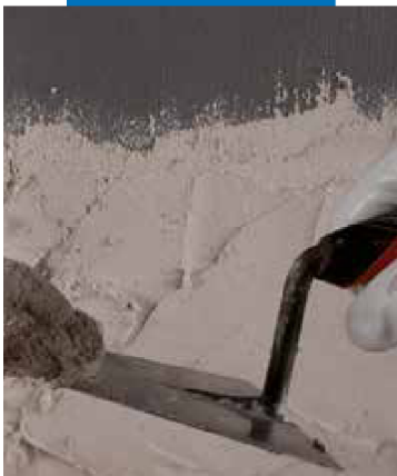
Application of render on Eco Prim Grip Plus
